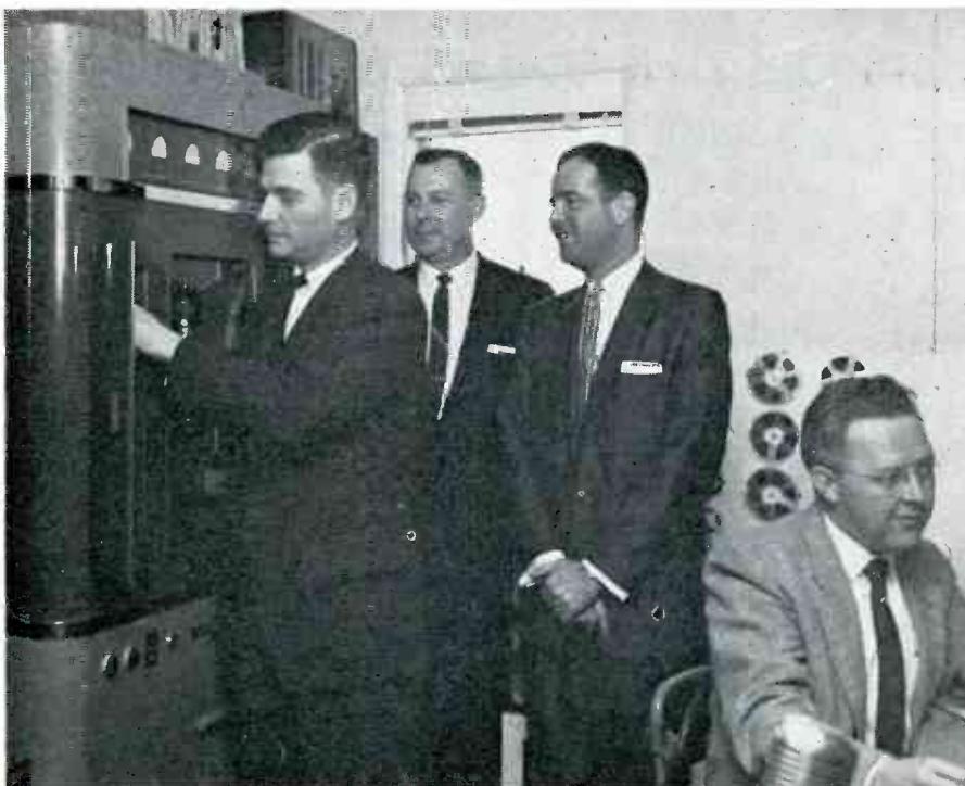
Governor Mark Hatfield of Oregon throws the switch at KPLK in Dallas, Ore., changing over from 500 watts to 1,000 watts on KPLK's 4th Anniversary. The Collins 550 A- Transmitter had been previously converted to a 20V-2 and operated at half power. The Governor is turning power switch to full power. (L. to R. are Gov. Mark Hatfield, Station Manager Ray Kozak, Gerry Frank, manager of Meier & Franks Store in Salem and seated is the chief engineer, George W. Morrison.)
